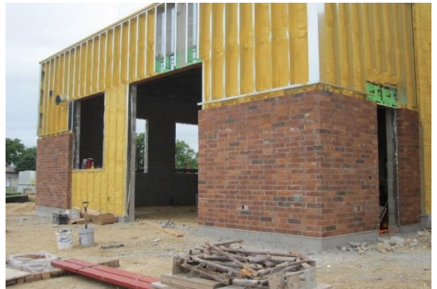
Brick veneer on the exterior of the addition, fiber cement panels on the upper walls will follow shortly
