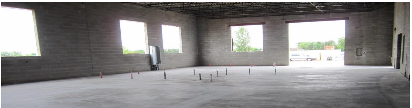
The cured concrete slab for the new metals lab shown above. The conduit stubs shown sticking from the slab will provide power to the welding booths.
