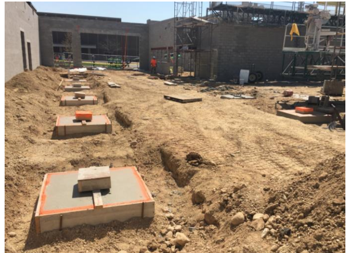
Column footings are completed and ready for steel erection!
