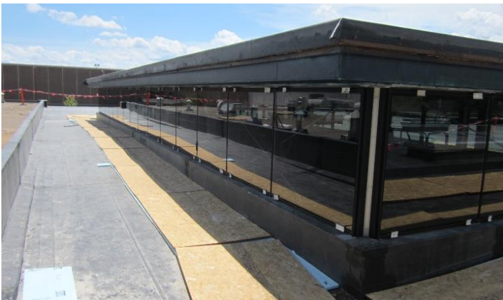
Glass has been installed at the clerestory
