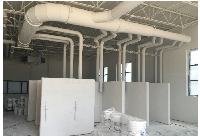
Painting has started in the shop spaces!
