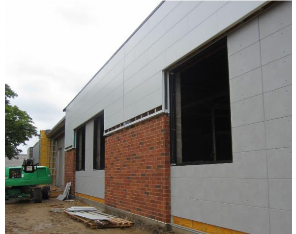
The "Nichiha" siding is being installed
