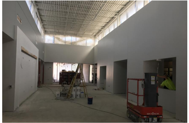
The new STEM space has been painted. Casework installation, MEP finishes, and ceiling installation will begin soon!
