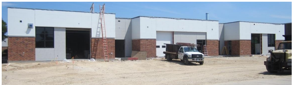
The exterior of the building is nearly complete – overhead doors have been installed, and "Nichiha" siding and exterior glazing are nearing completion! Site grading has begun in preparation for paving.
