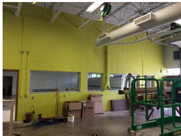
The freshly painted walls and ceilings in the construction lab.
