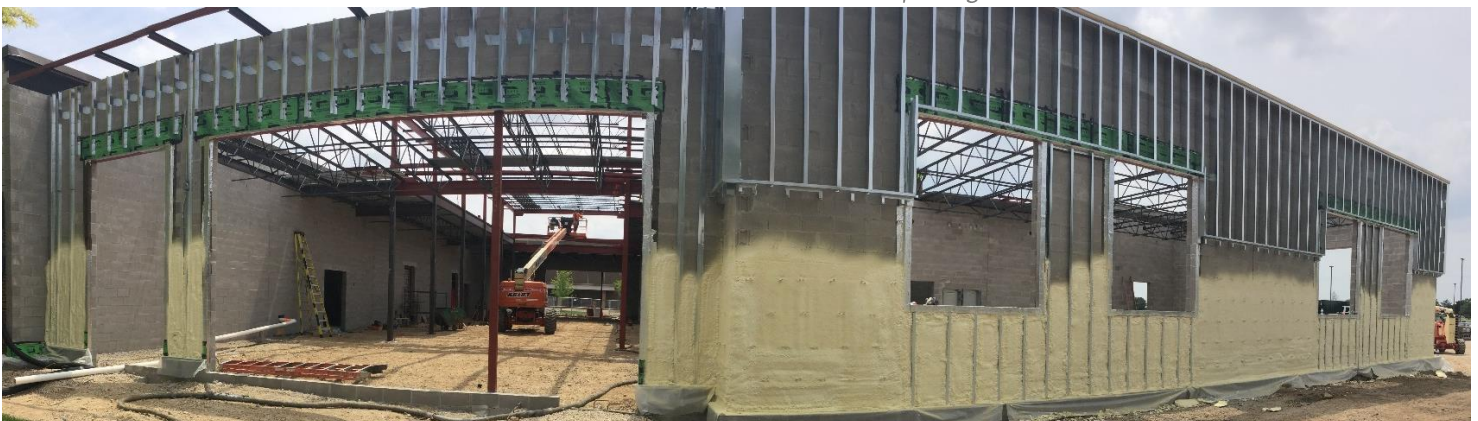
Spray foam insulation has been applied to the north elevation
