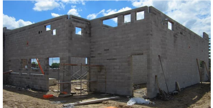
Load bearing masonry walls are topped out!
