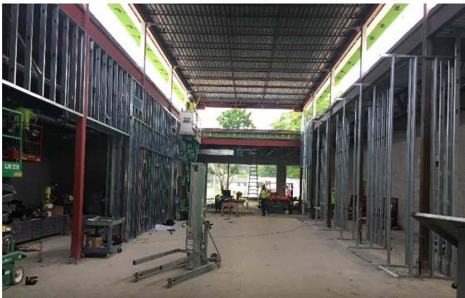
Wall framing has begun, and the building is taking shape. After the MEP trades have installed their rough-ins in these walls they will be ready for drywall!
