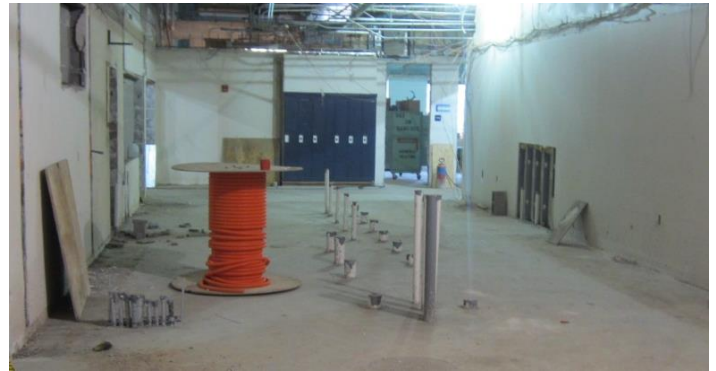
The existing concrete floors were cut open to allow new plumbing work to be installed underground before being backfilled and infilled with concrete. All of the pipes shown here will serve future bathroom fixtures
