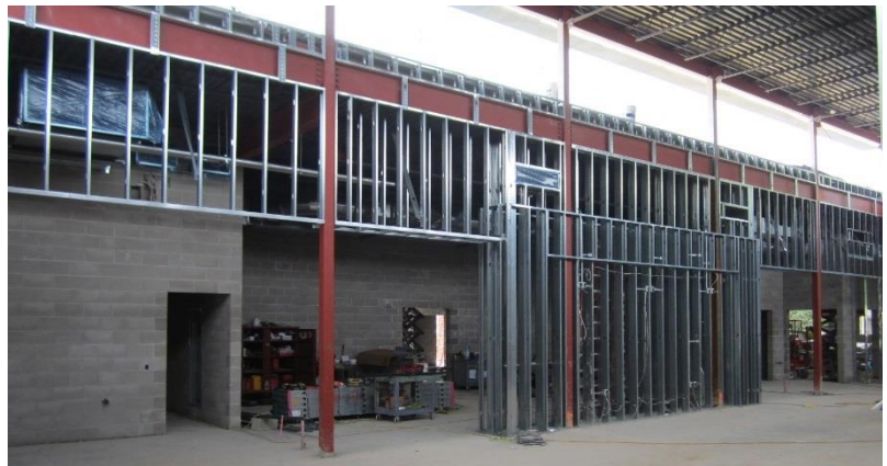
Wall framing has begun, and the building is taking shape. After the MEP trades have installed their rough-ins in these walls they will be ready for drywall!
