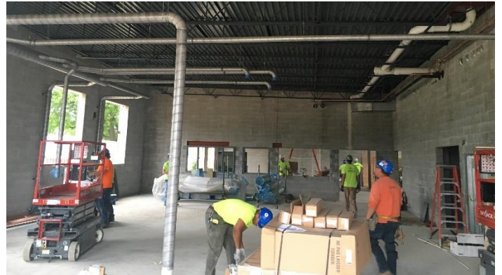
HVAC, plumbing and electrical crews are working to get ductwork, piping and conduit installed in preparation for painting
