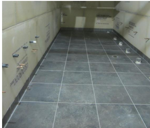
Finishes are now progressing into the existing building – bathroom tile floors have been installed, and drywall is being taped and finished in preparation for paint!
