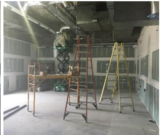
Finishes are now progressing into the existing building – bathroom tile floors have been installed, and drywall is being taped and finished in preparation for paint!
