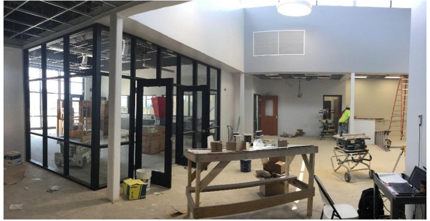
Interior storefront glass has been installed in the STEM area!
