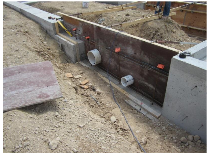
The stubs of piping in the wall have been installed to facilitate the future installation of underground plumbing work.
