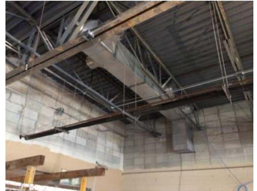
New duct work is installed for the new air handling unit that serves the remodeled STEM lab.
